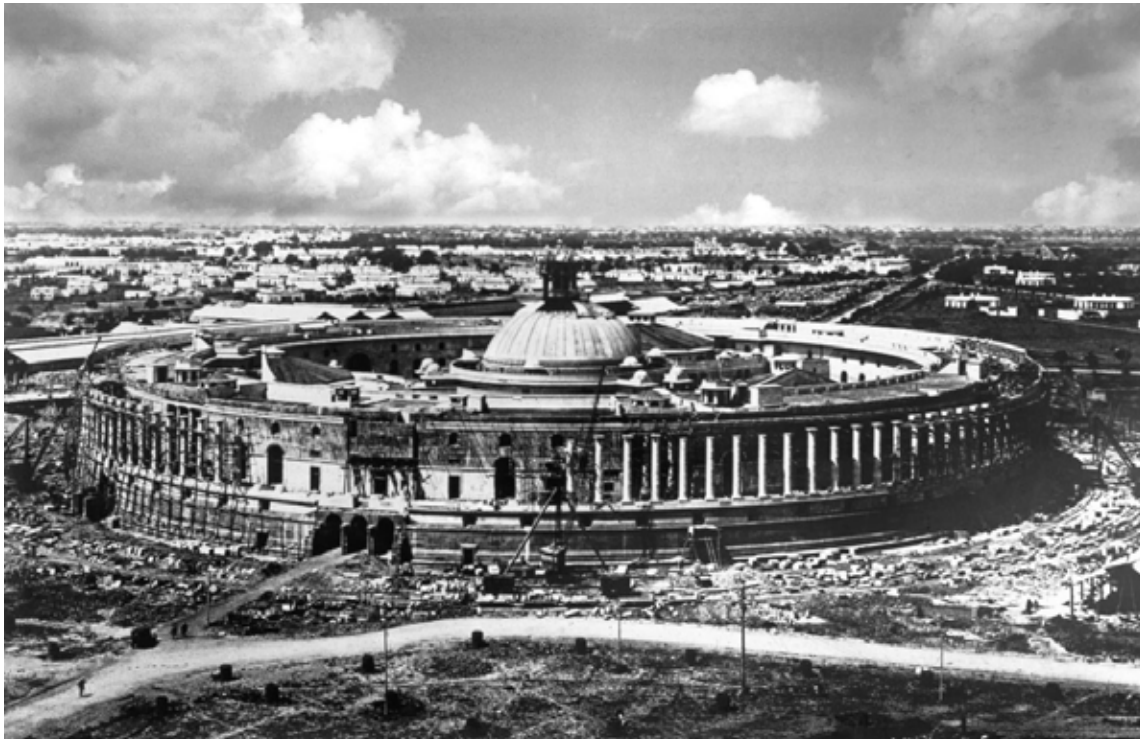
▲ Parliament House under construction
